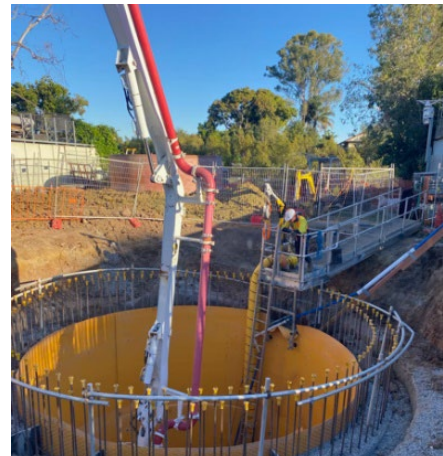
Frederick Street - Wet Weather Pump Station at 10m in depth
