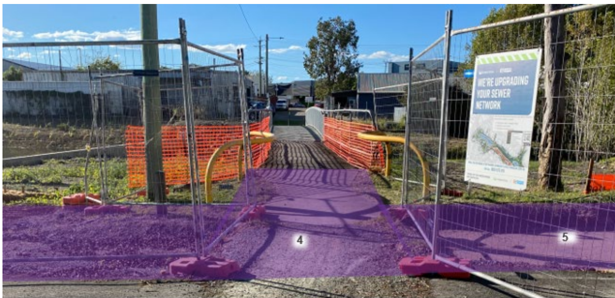
Image 3: Access to the pedestrian bridge
