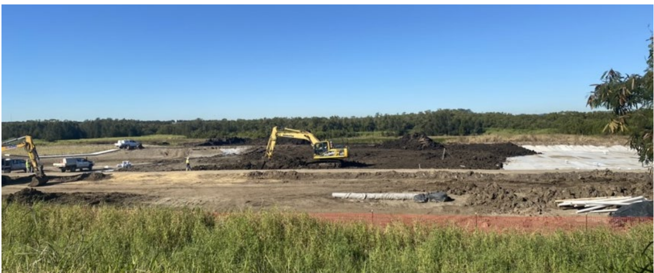
Image 8: Bio-retention basin Southern Cross Way - placement of topsoil
