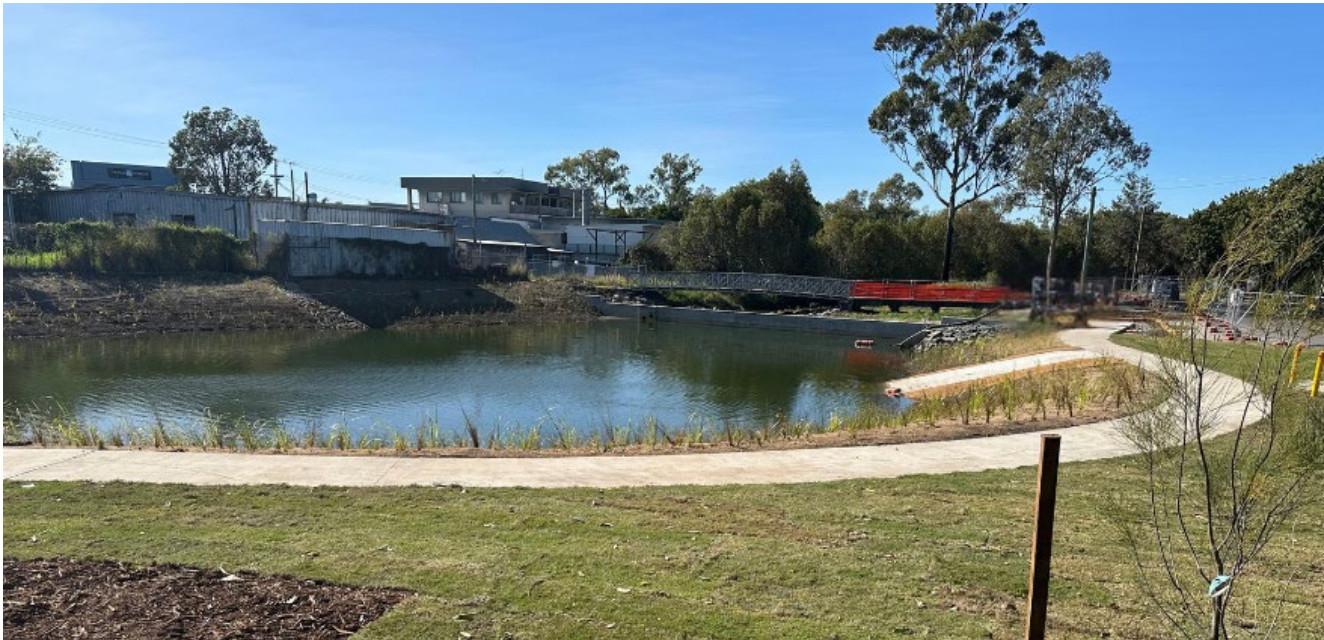
Image 1: Sediment basin one at Station Avenue – 4 June 2025
