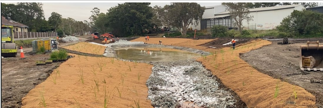
Image 6: Sediment basin two at the end of Carter Street facing north
