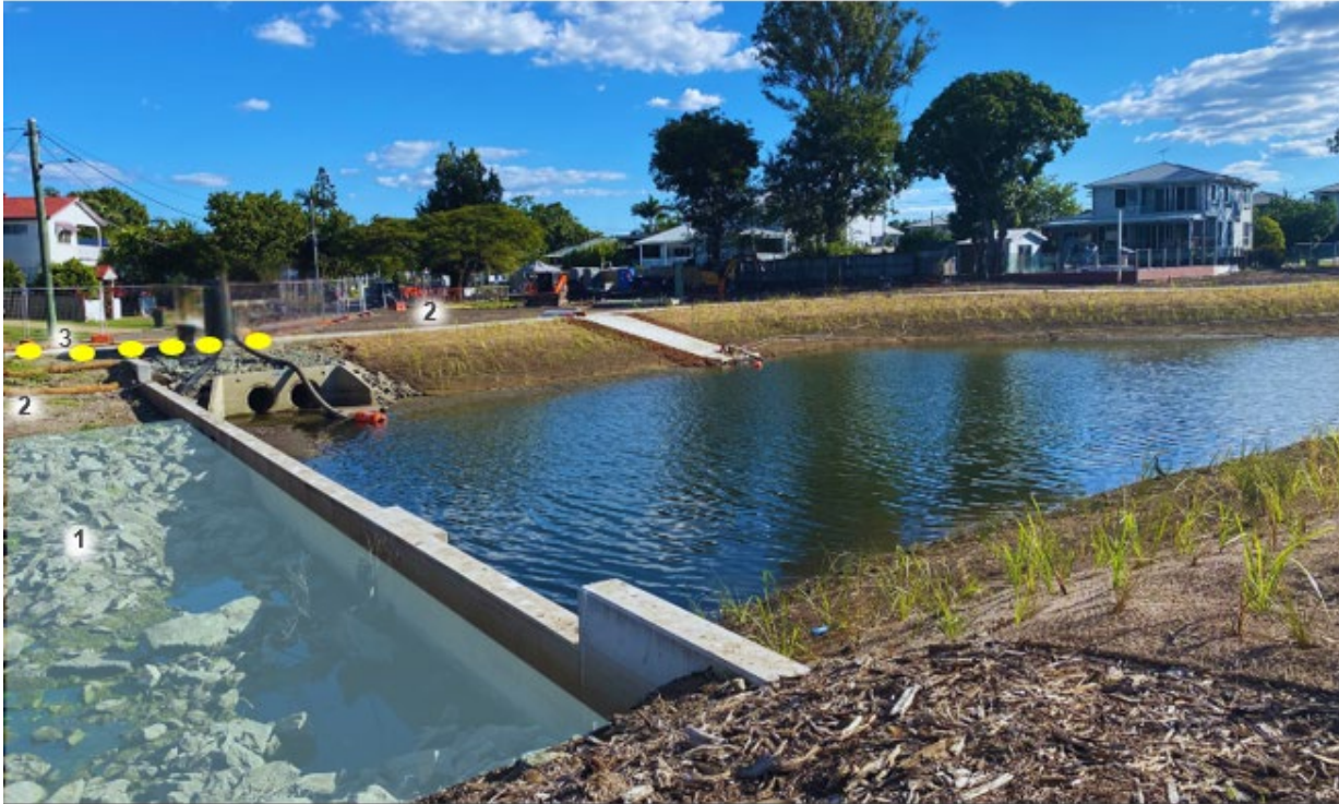
Image 2: Sediment basin one at Station Avenue
