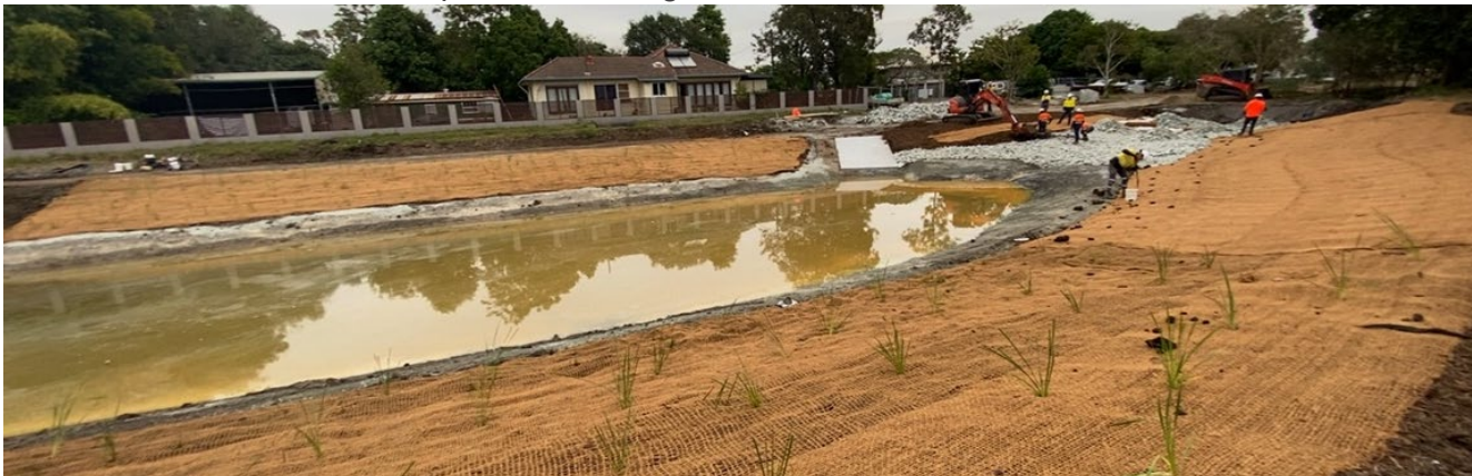
Image 5: Sediment basin two on northern side looking towards Carter Street
