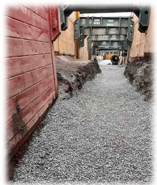
Image 2: Shore box installed in the trench
