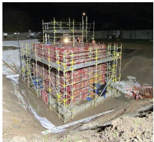
Expedited screening chamber base poured and wall starter bar
